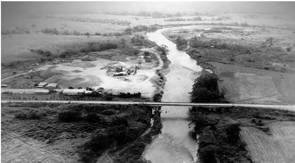
The Pacora River bridge
