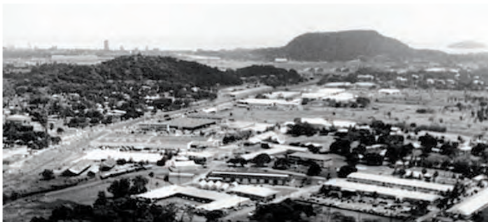
Ancon Hill ( right ) as seen from the vicinity of Fort Clayton, the location of JTF-South's operations center
