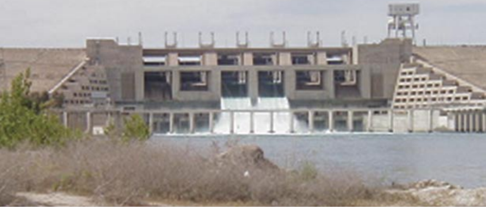
The multilevel Hadithah Dam complex houses six large generators and six turbines, which provide electricity to the surrounding region
