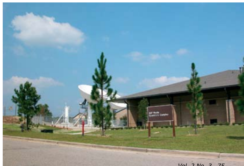
The USASOC Media Operations Complex at Fort Bragg.
