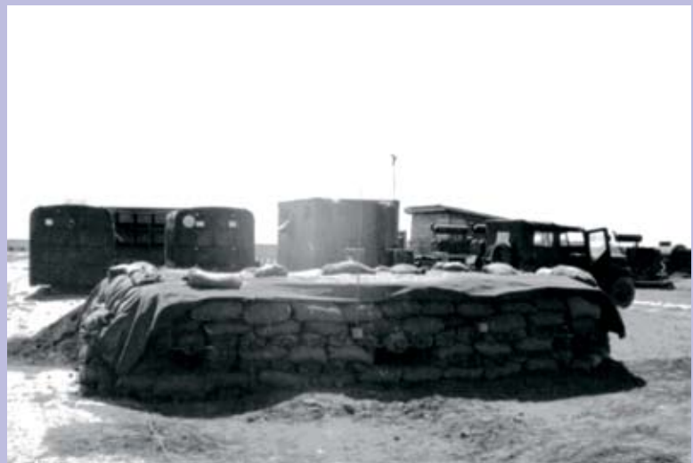
Team bunker being built at the radio station. This is the bunker where the team gathered during the attack.
