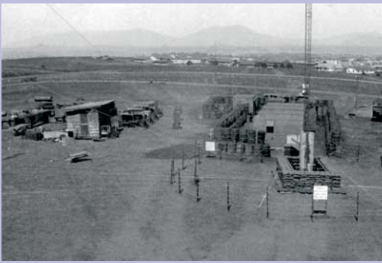
View of the completed radio station from the guard tower. The TRT-22 transmitting modules are in the center of the stacked 55-gallon drum barrier. The 250-foot antenna base is clearly visible. To the left of the photo are the generators and the generator mechanic's shed.
