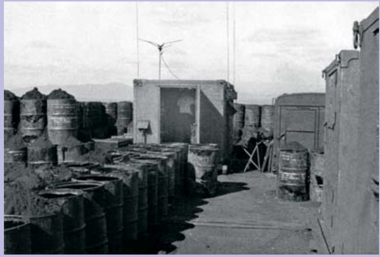
View of the force protection for the radio system. The 55-gallon drums were filled with dirt. Two rows of drums served as the base with a third row on top to protect the facility from rocket and mortar fire.
