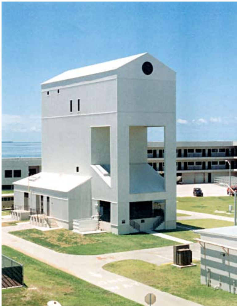
The new fifty-foot dive tower allows for the simulation of locking out of a submarine and for training in the free ascent from deep water.
