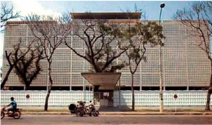
The American Embassy in South Vietnam was located on Thong Nhut Boulevard in Saigon.
