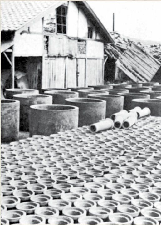
Cement donated by UNCACK was used to make culverts and well casings in July 1952. As the war grew static, UNCACK's mission shifted to that of helping rebuild the South Korean economy.
