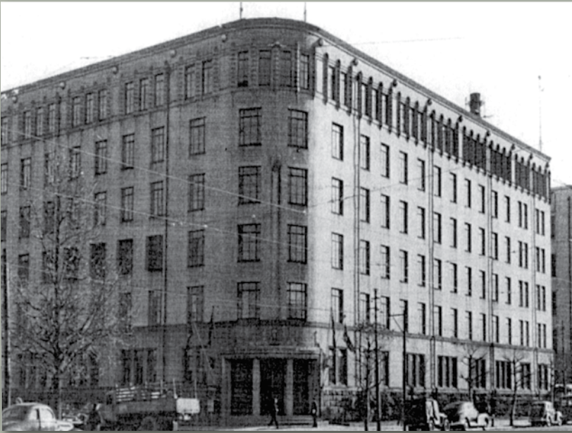
The 1st RB&L headquarters occupied the sixth floor of the Empire Building on Avenue A in Tokyo.
