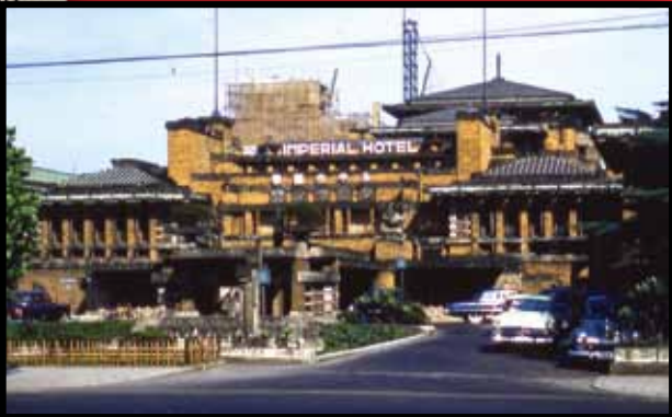
Imperial Hotel designed by Frank Lloyd Wright. Photo taken during the Korean War reconstruction period 1953-54.
