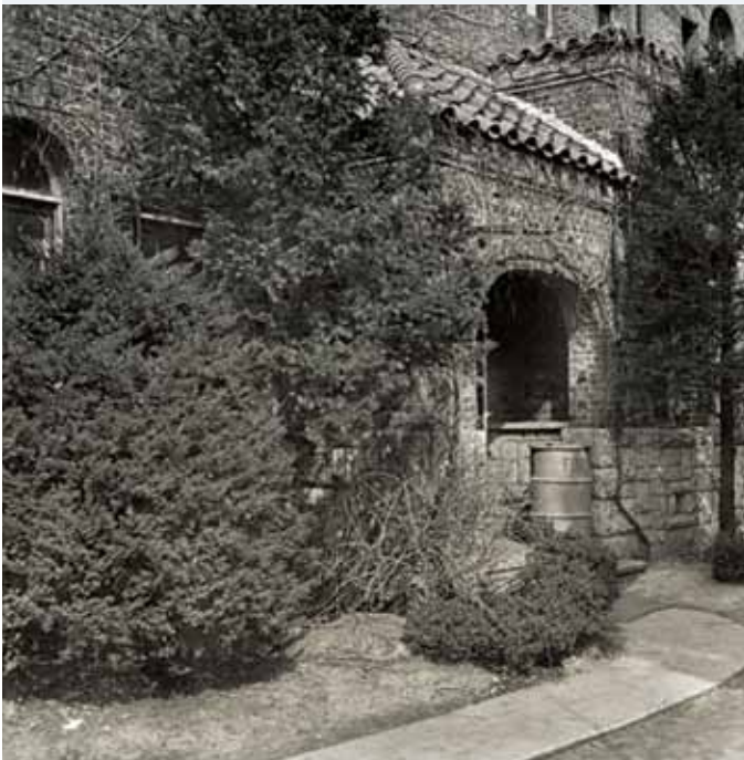
FEC/LD (K), at first independent from CCRAK, was later a subordinate unit. Its headquarters in Seoul, pictured here, was near that of CCRAK.
