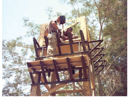
Figure 9.17 Construction of guard tower platform skirts.
