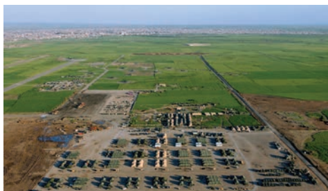
Figure 7.24 Aerial view of Camp Loki.
