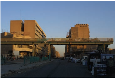
Figure 8.13 Crosswalk vantage point. This elevated crosswalk is where the Iraqi gunman ambushed the Civil Affairs public health team convoy.
