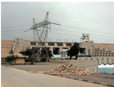
Figure 7.52 Power lines at Haditha Dam. The multilevel Haditha Dam complex houses six large generators and six turbines, which provide electricity to the surrounding region. Only one was fully operational when the Rangers seized the objective.
