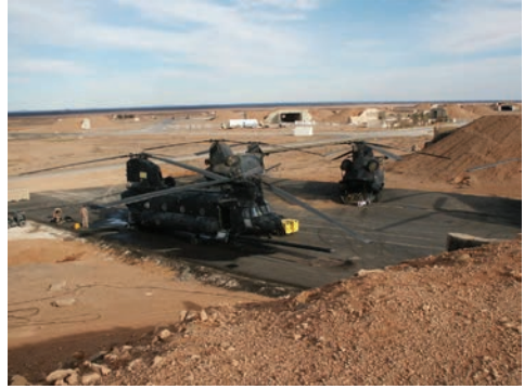
Figure 4.17 Pad at H-5. With the pad in place, the helicopters of the 3rd Battalion, 160th SOAR, were able to rapidly prepare for missions.
