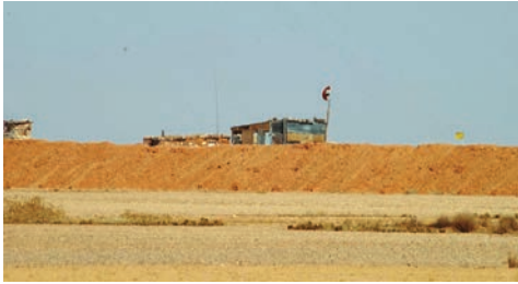
Figure 5.50 VISOBs building. Most of the Iraqi visual observation posts were destroyed in the first night of operations, effectively blinding the Iraqi higher command.
