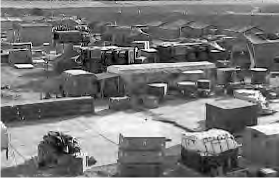
FIG 35. K2 buildup with backlog of accumulating supplies and equipment.
