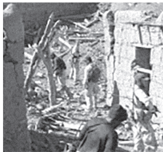
FIG 9. Babulkhel damage assessment.
