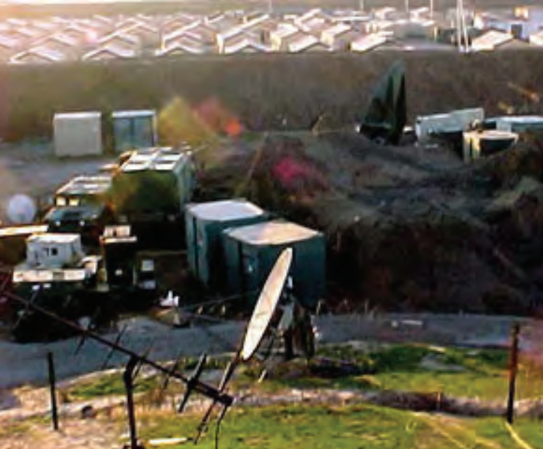
FIG 54. Antennas, power, and cabling were installed first.
