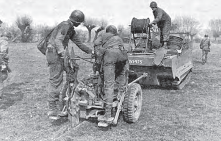
Unidentified WWII signalmen bury spiral-4 cable near the Rhine River.
