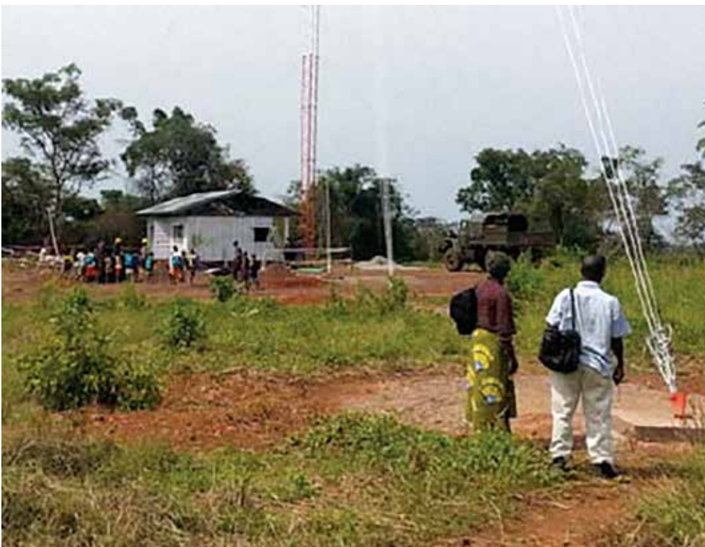
A view of the radio station and antenna in Djema months after installation.
